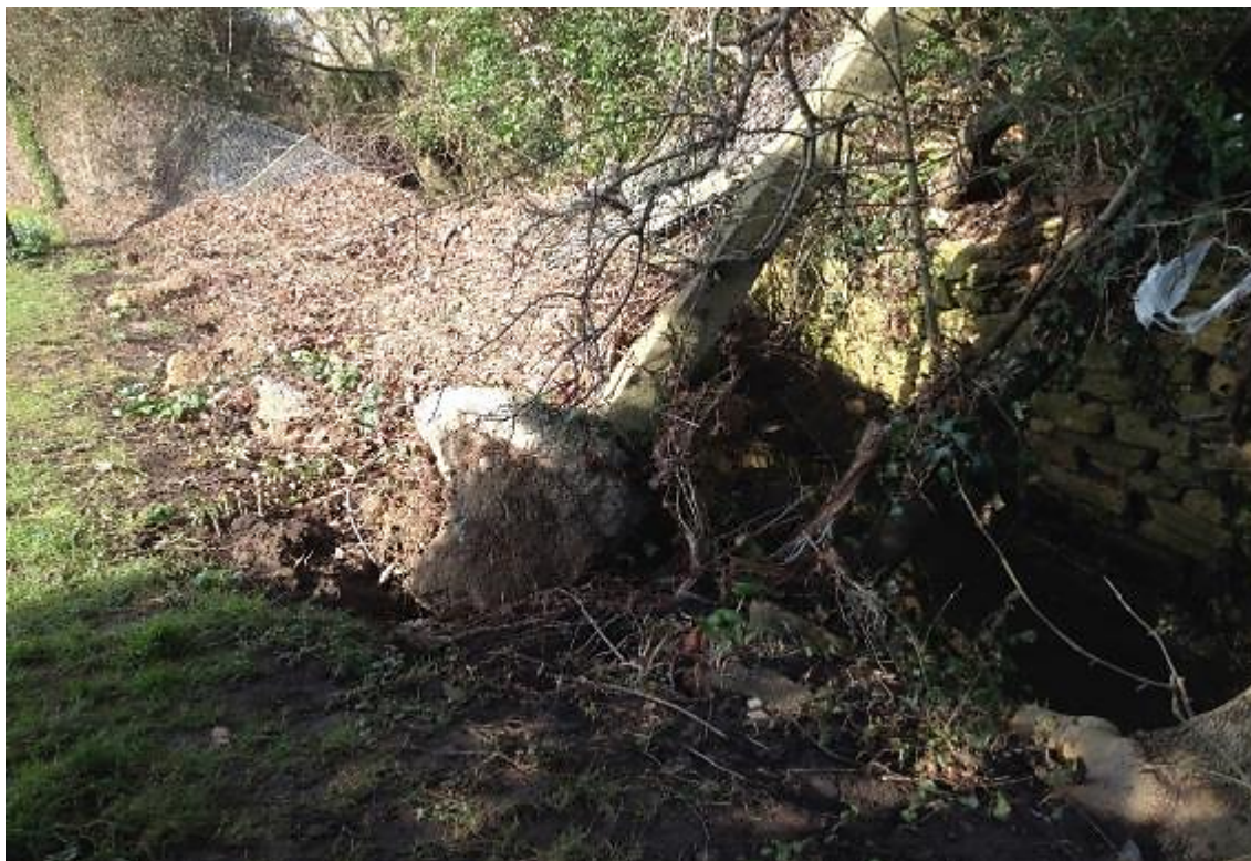
Fig. 5 Martock Recreation Ground - damaged chain link fencing on 06.02.16
