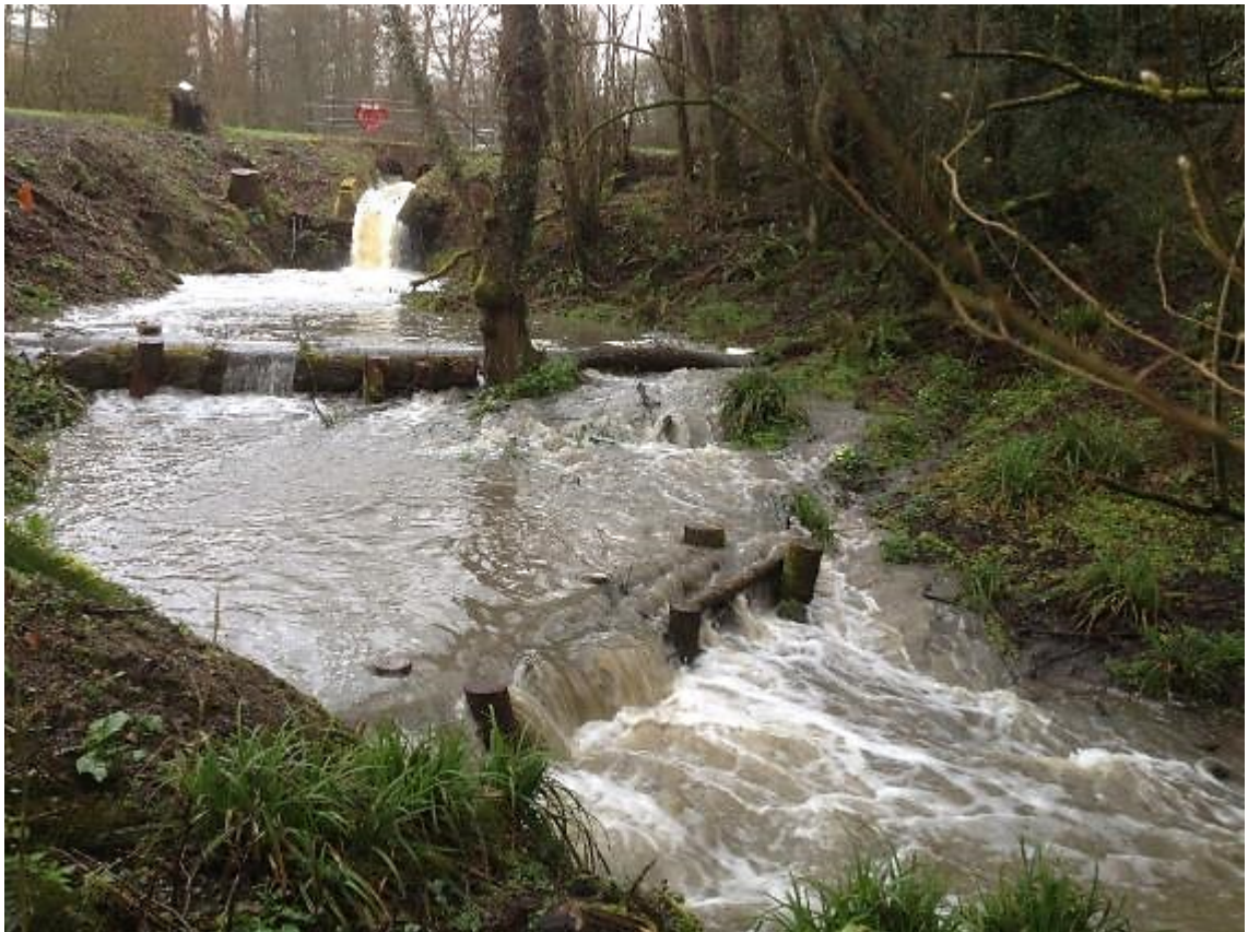
Fig. 8 Release of flood water at Lufton, 31.03.18.to create storage for rainfall 01/02.04.18
