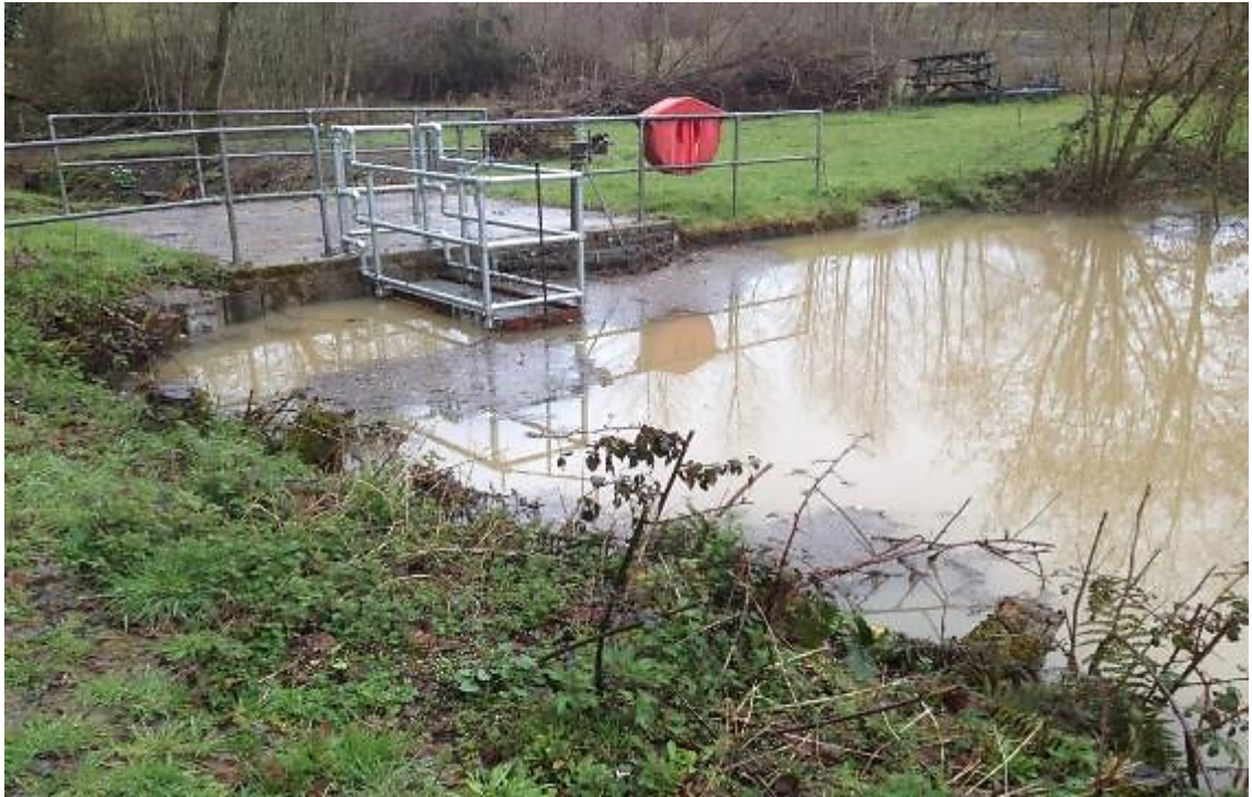
Fig. 7 Flood storage at Lufton – full on 31.03.18
