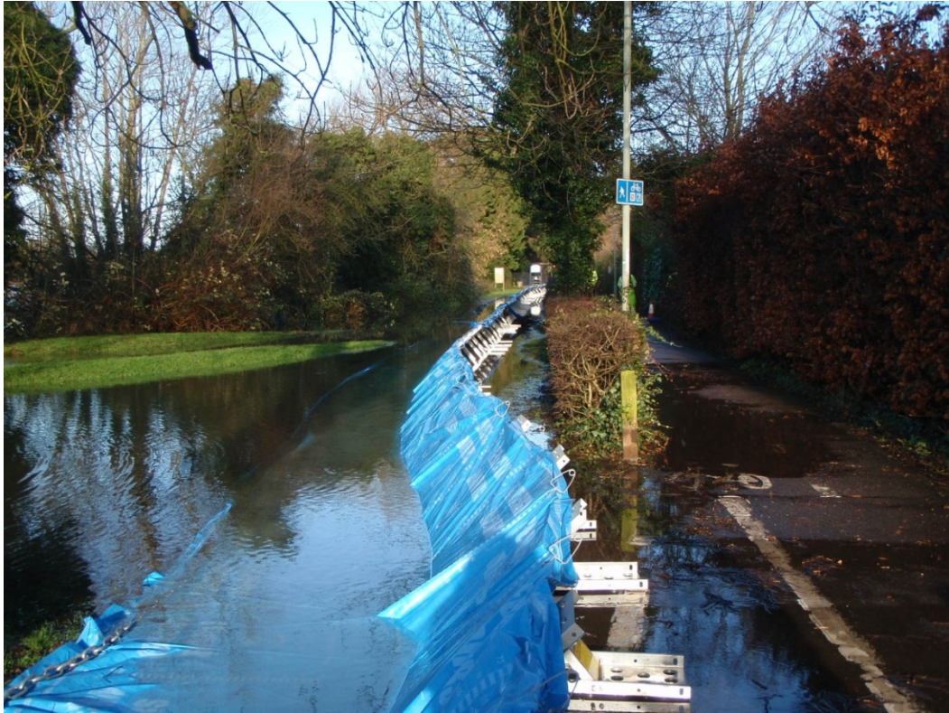
Figure 9: Temporary defences deployed in Oxford in January 2014.
