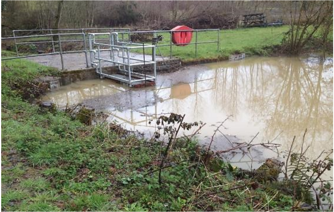
Fig. 7 Flood storage at Lufton – full on 31.03.18
