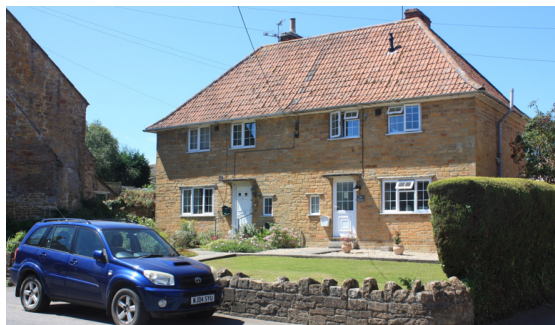
This pair of stone Petter and Warren houses is one of several built in Bower Hinton between the wars.
