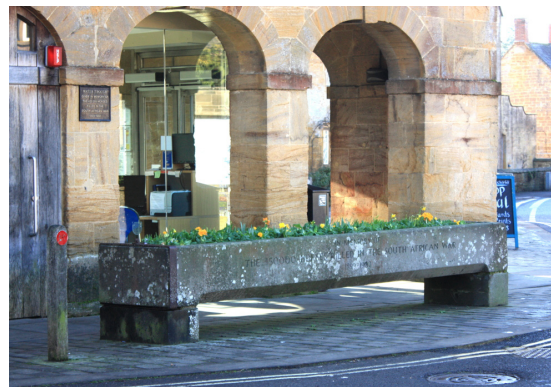
Next to the Market House (now the Parish Office) is a House Trough, once a functional one at the railway station. One purpose is indicated by its inscription, 'in memory of the 150,000 horses killed in the South African War'
