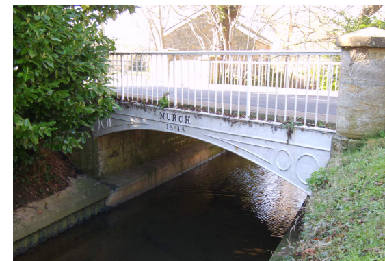
The grade 2 listed Hurst Bow Bridge from the Martock side. Made in 1843 in cast iron by Edward Murch, an ironfounder in Bridgwater. The other side of the bridge is Hurst.
