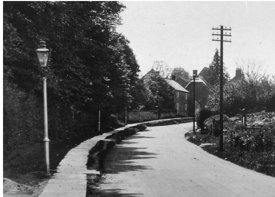
The blue lias raised pavement of Bower Hinton in the 1930s. The walls still exist and are an important village feature but the tops are now mainly asphalt and the individual house access steps have sadly largely been sacrificed to the car.
