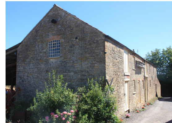
This is the barn and dovecote of Bower Hinton Farm. It is a typical functional nineteenth century Martock building. The cast iron window frames, segmental arched brick doors and window lintels and the pulley wheel in the apex to drive external machinery, all betray the Sparrows Foundry influence that pervades Bower Hinton.
